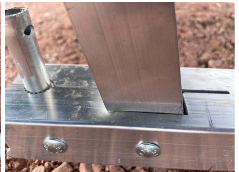
PHOTO 15: Upright deformation after testing
