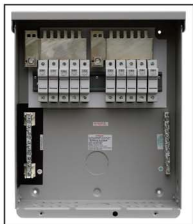
MNPV12 Configured for 600VDC fuses (Gridtie)
