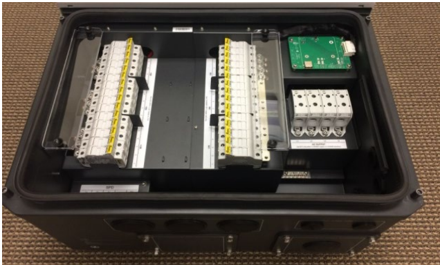
Figure 10-1 Remove Wire Box Cover
